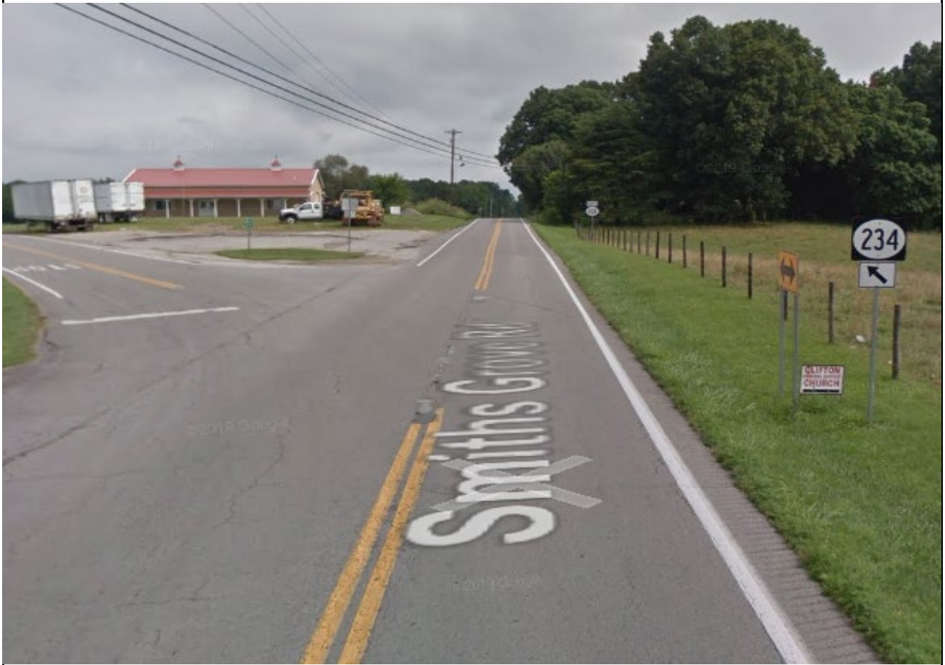
Photo 1: Beginning of the project at the KY-234 intersection facing north toward Warren County
