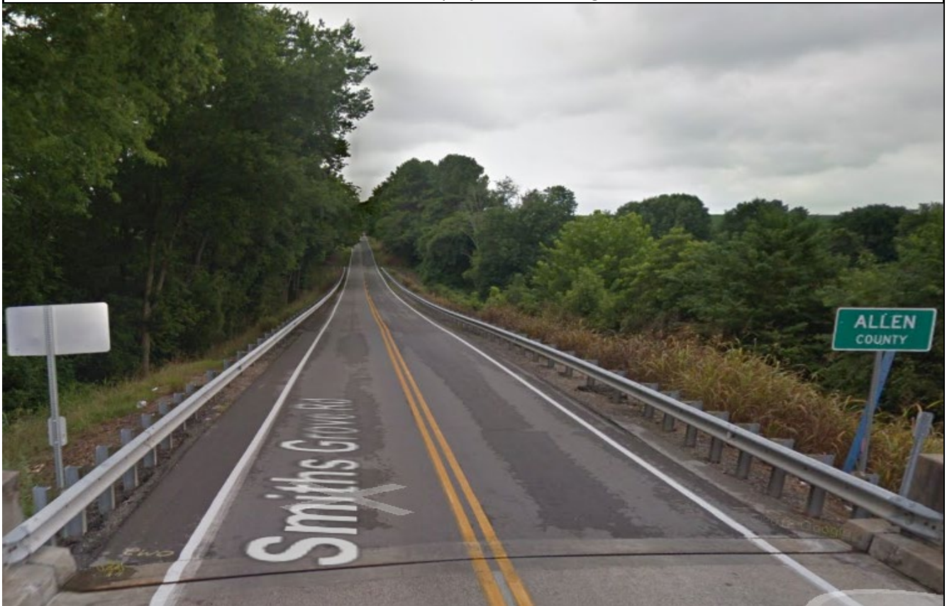
Photo 4: End of the project at the Warren County Line facing south toward Scottsville
